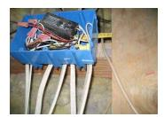
An electrical connection has been incorrectly made outside of a junction box, which is a potential fire-hazard. All such connections should be made inside a junction box, in order to contain any arching or sparking within the box.
