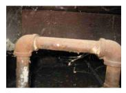
Gas SupplyPipes Components and Conditions Needing Service Rust has been noted and should be watched.
